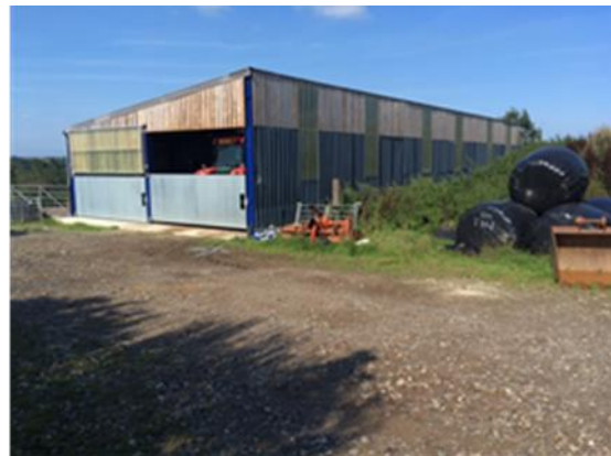
Existing agricultural building (views to south and east)
