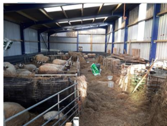
Buildings used for lambing/machinery storage
